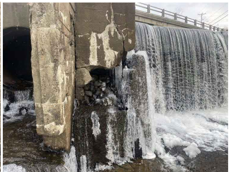
November 2021 – Dam to concrete structure
