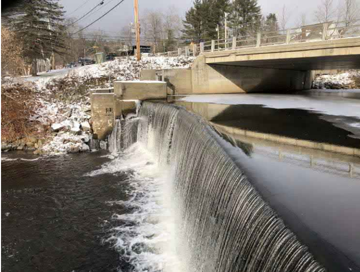
November 2021 – Primary Spillway
