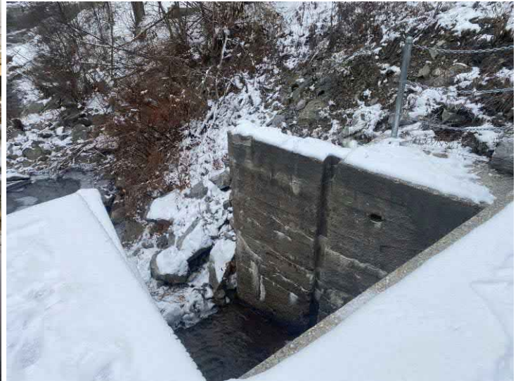
November 2021 – Right wall of Outlet Flume
