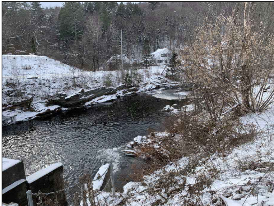
Downstream side of the dam, looking south from N Main St.
