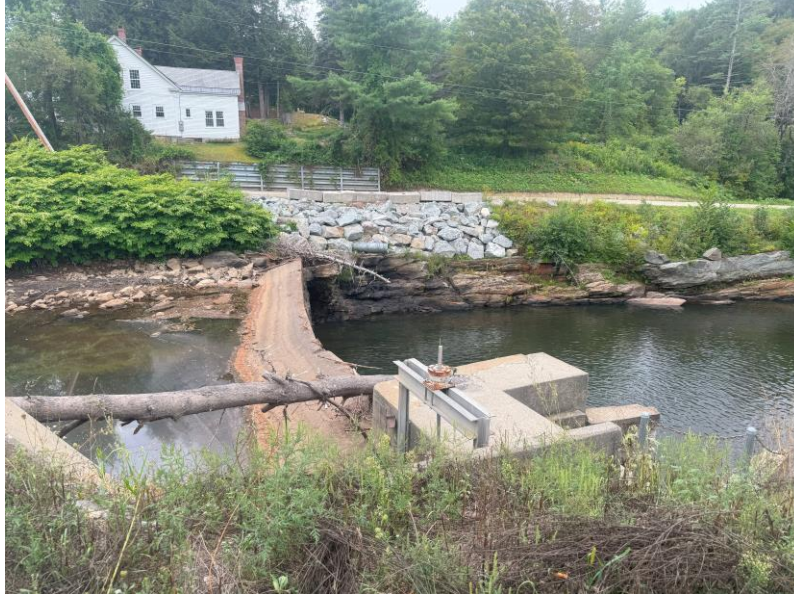
Photo 1. Concrete sluiceway structure viewed from right abutment of dam
