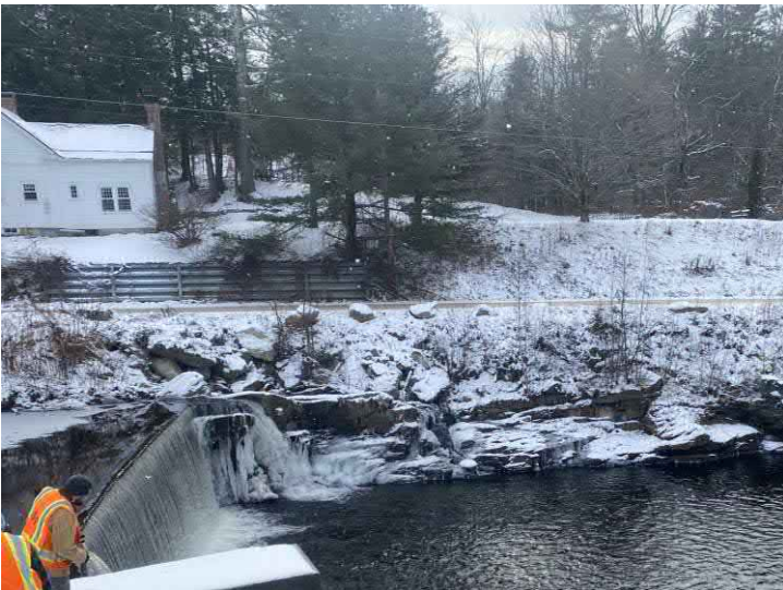
November 2021 – Left Abutment
